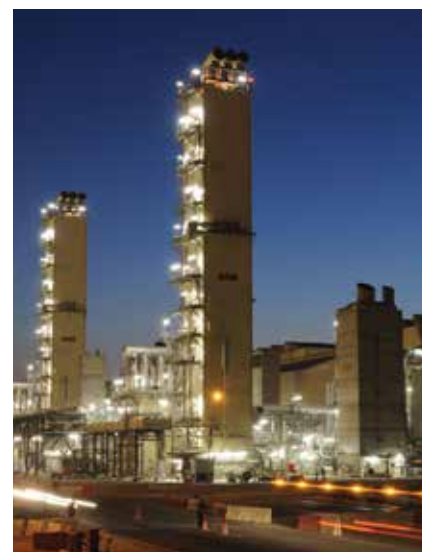
PEARL GTL, QATAR
