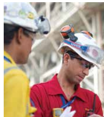
PEARL GTL, QATAR
